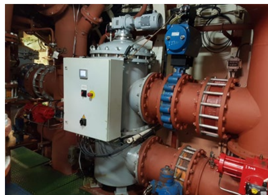
Ballast water treatment system, Algoma Integrity
