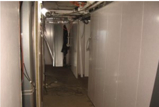
Lining installation for accommodations.
