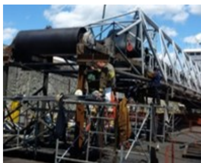
Algoma Enterprise - boom repairs underway (L) and boom hood deflector repaired and ready to be returned (R).
