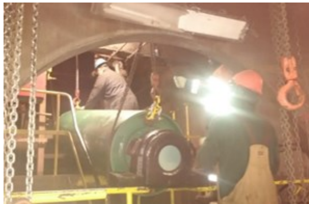
Replacing an Inner Loop Pulley on the Algolake .
