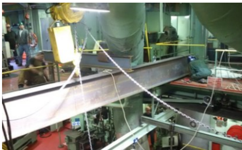
Above: Installing lifting beams in the Engine Room on the Captain H. Jackman to remove Crank Shaft.
