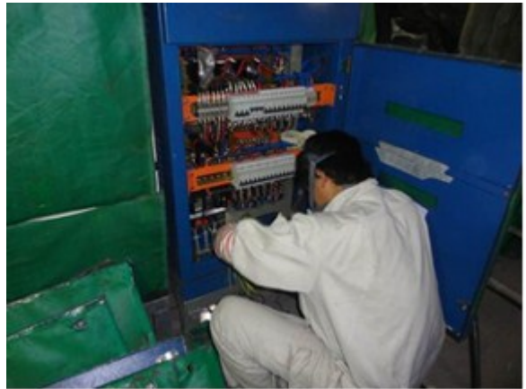
Equipment cable termination in Engine Room.
