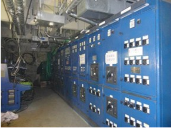
Main switchboard in Engine Control Room.
