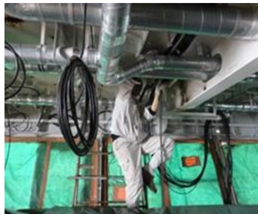
Cable pulling in accommodations.
