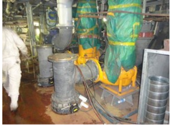
Fresh water cooler outfitting.
