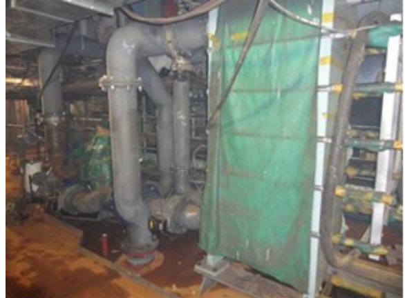
Lube oil cooler outfitting.
