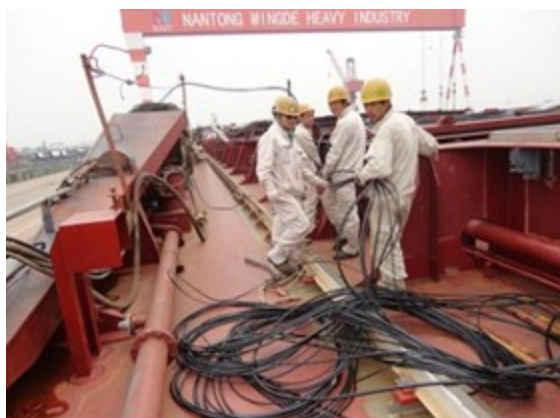
DVS installed, cables being pulled.
