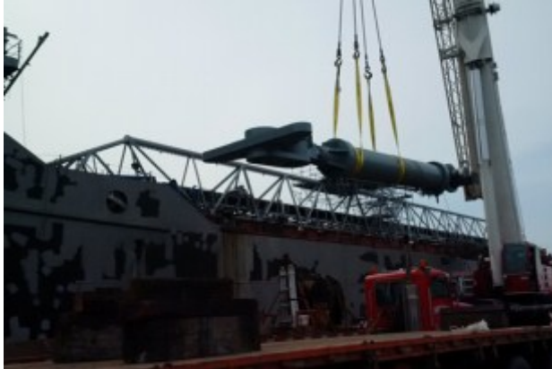
Removal, overhaul and re-installation of Boom Luffing Cylinder and Boom Link Assembly.
