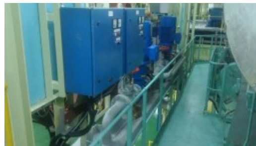
Completed installation of Xhead pumps, piping and cabinets aboard the Algoma Equinox .
