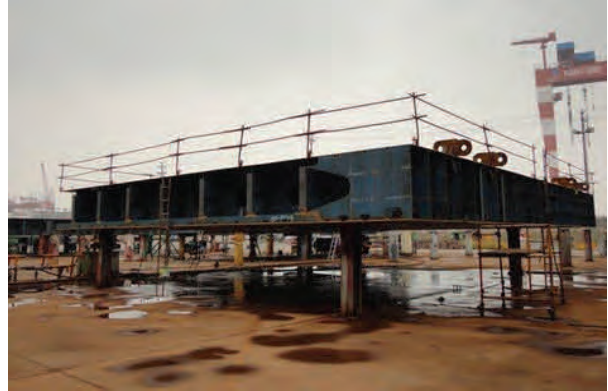
Hull 153, 1 st Self-Unloader, Midship DB Block
