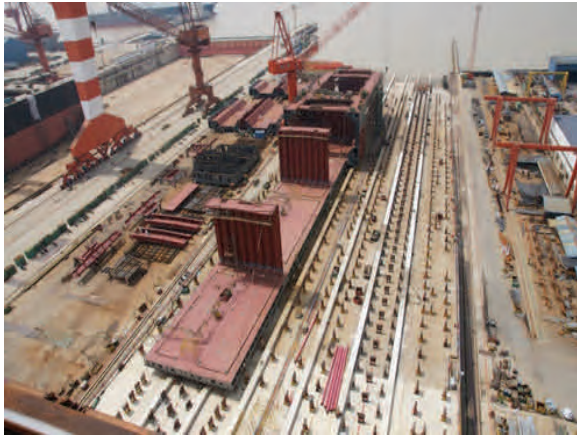
Side tank blocks being erected with cross decks
