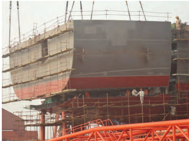
Final main hull block being installed.
