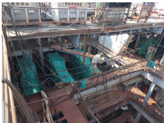
Auxiliary Generator installation in Engine Room
