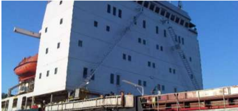
The new boarding ladders installed on the Algoma Guardian.
